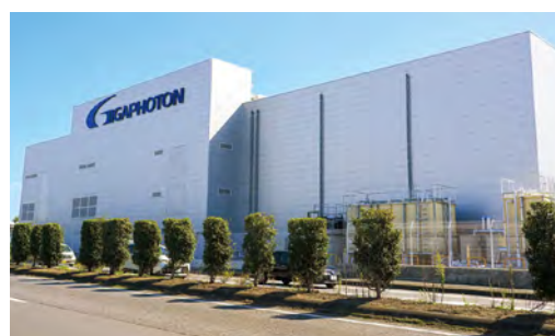
[Gigaphoton Inc.'s new production building]
