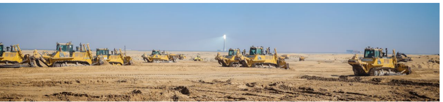
Leveling trial with ICT bulldozer
