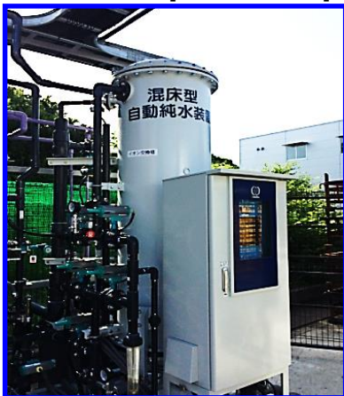
Water purifier for process water
