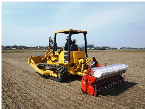
Direct seeding by multifunctional ICT-intensive dozer (Reduced man-hours and machine expenses)
