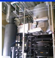
Biomass boilers at the Awazu Plant and wood chips
