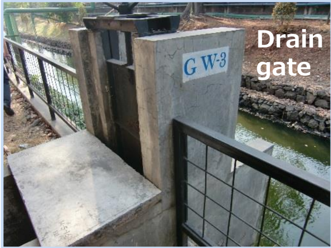
Indonesia (KI) : Measures against flood
