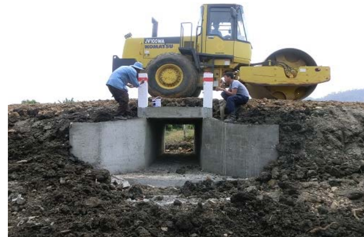
Box culvert (small)
