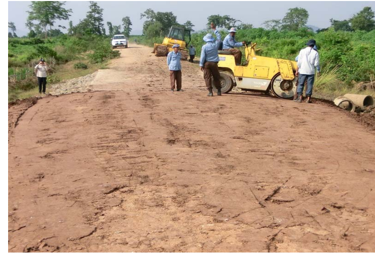
Restoration work completed
