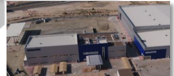
Dubai Training & Demonstration Center in UAE
