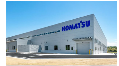
Seal ring factory at Himi Plant
