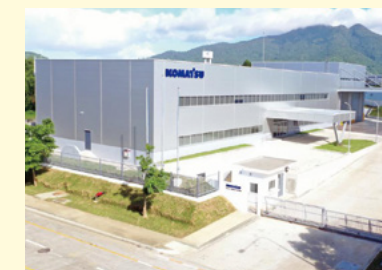
New building of Komatsu Philippines Corporation
