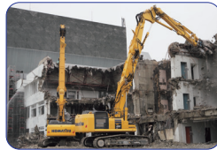
High reach demolition
