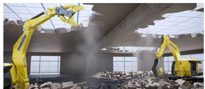
Fig. 11 An example of use at an indoor demolition site (CG)
