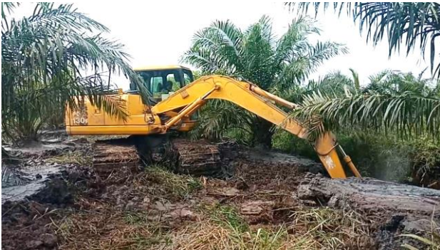
Fig. 19a Scene of actual operation (water channel maintenance)
