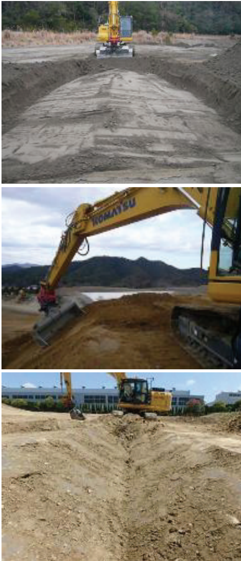
Fig. 9 Result of Construction Using Auto Tilt Bucket
