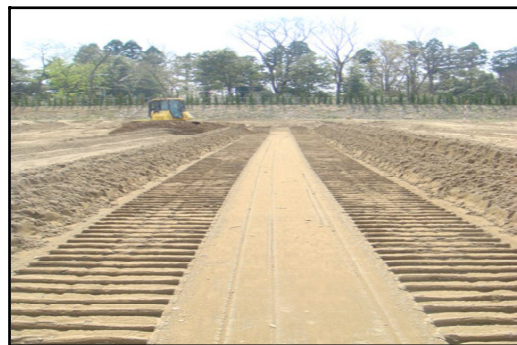
Fig. 14 Leveling accuracy and execution plane by leveling work execution by IT design
