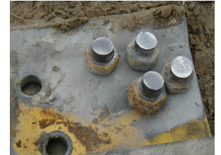
Photo 6 Fallen shoe, bent bolt
