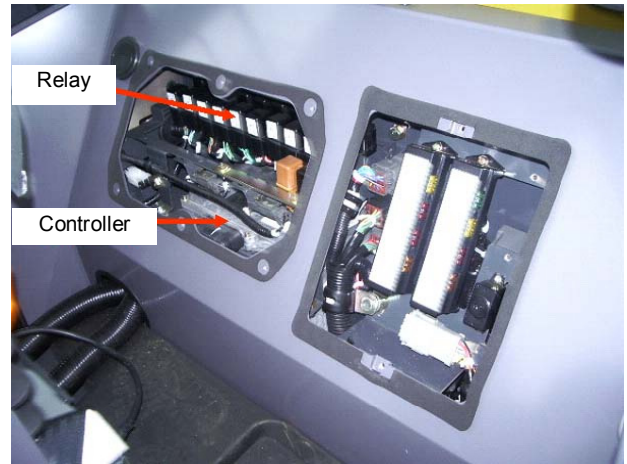
Fig. 18 Waterproof box inside cab
