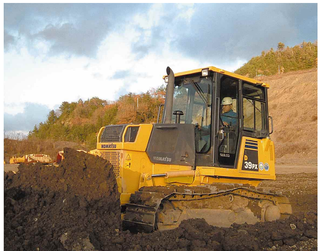
Photo 1 General view of D39PX-21
