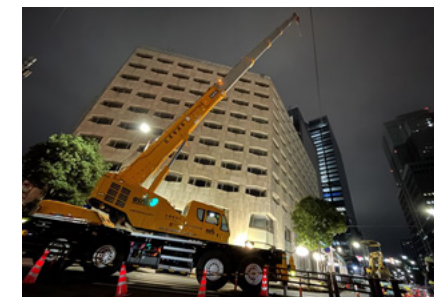
Trees being removed by crane
