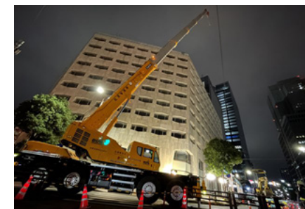
Trees being removed by crane
