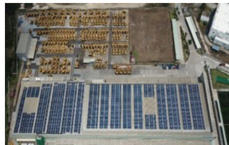
Solar roof installed in FY2018
