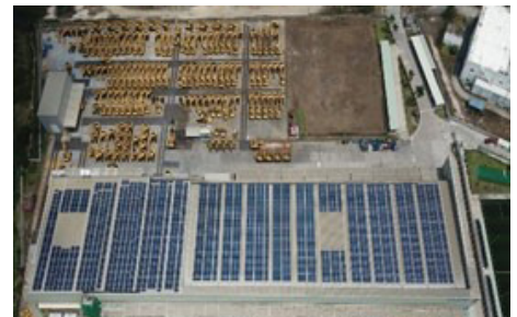
Solar roof installed in FY2018
