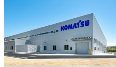
Seal ring factory at Himi Plant
